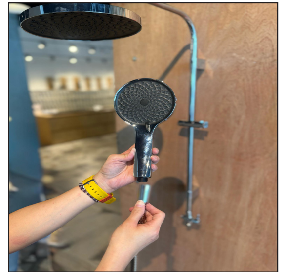
Step 12: Before attaching the handshower, ensure the O-ring is properly seated on the 1.5m hose for a secure connection.
