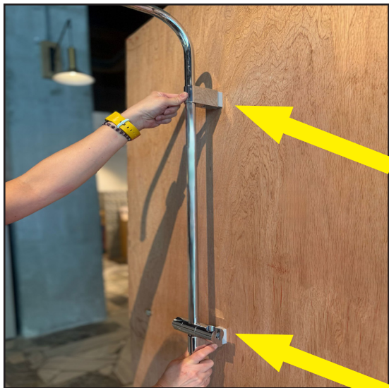
Step 8: Attach the shower rod to the wall bracket until it clicks securely into place
