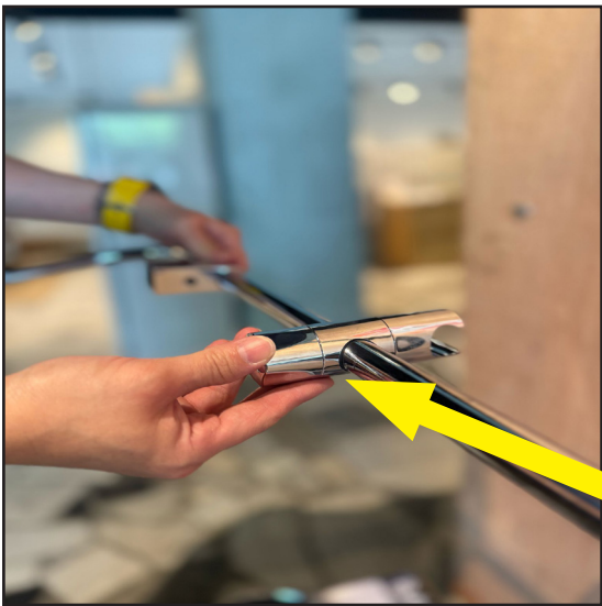
Step 7: Use Allen key, turn anti-clock-wise to tighten connector nut.
